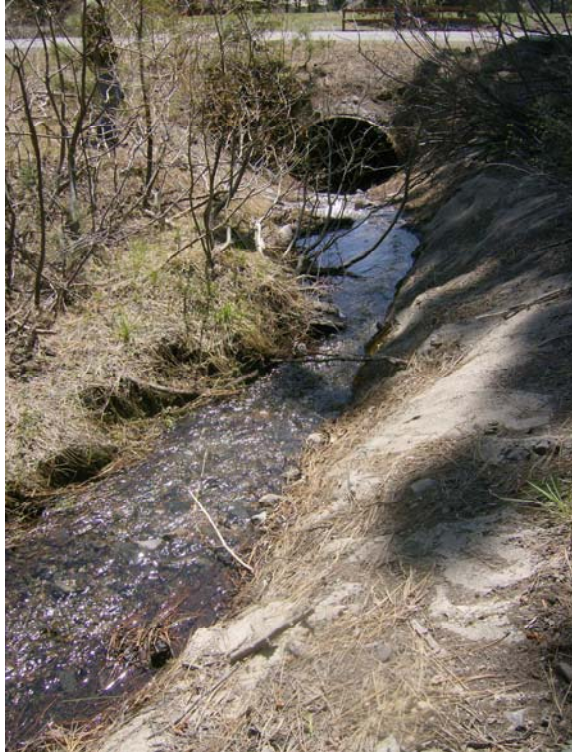
PP3: Lake Forest Creek flowing through culvert beneath SR 28, Facing South
